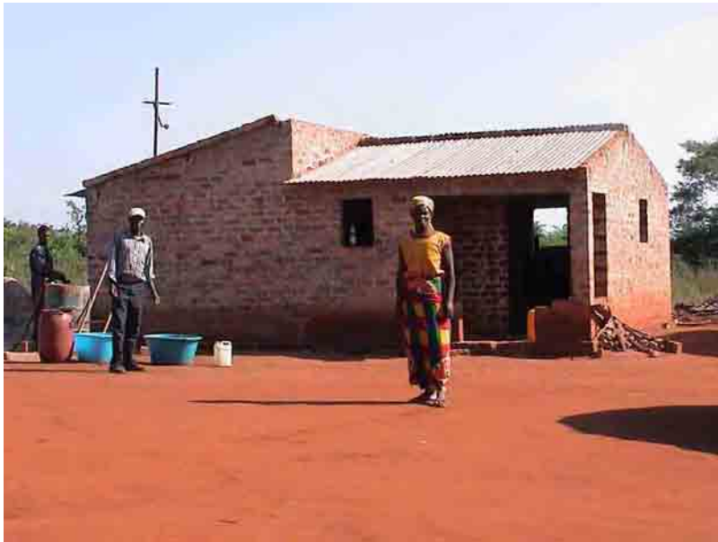
Building For VitaGoat Production
